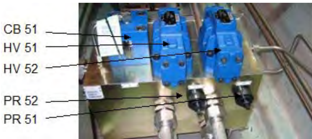
Figure 40. Adjusting the pressure relief valve PR51
