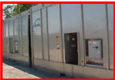
91345 Marley, NC8307M1SS, 1950 GPM, 60 HP
