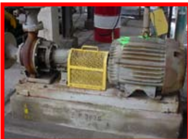
90773 Durco, Mark II, 450 GPM, 4" x 3" x 10"
