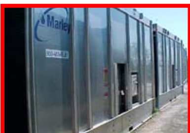
91369 Marley, NC8307M1SS, 1950 GPM, 60 HP
