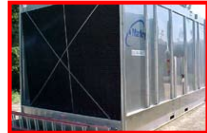
91368 Marley, NC8307M1SS, 1950 GPM, 60 HP
