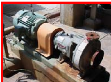
89464 Durco, Mark II, 90 GPM, 3" x 1.5" x 10", 20 HP, 203 ft head
