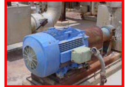
86521 Worthington, D1011, 1000 GPM, 8"x6"x13", 125 HP, Acero Inoxidable 316
