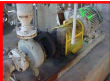
90788 Durco , Mark II, 190 GPM, 3" x 2" x 7", 15 HP, 150 ft head
