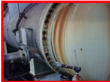
90971 Cust-O-Fab, 5981 pies 2 , 316LSS/316LSS/ CS, 75/75 psi, 450/200°F, Tipo BXM
