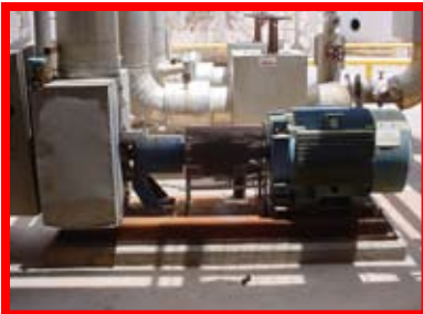
86520 Worthington, D1011, 1000 GPM, 8"x6"x13", 125 HP, Acero Inoxidable 316
