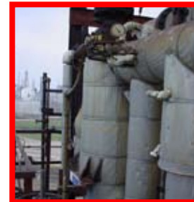
90975 Cochrane, 50 pies 2 , 304SS/304SS/ CS, 15FV/75 psi, 200/200°F, Tubos de 16 BWG
